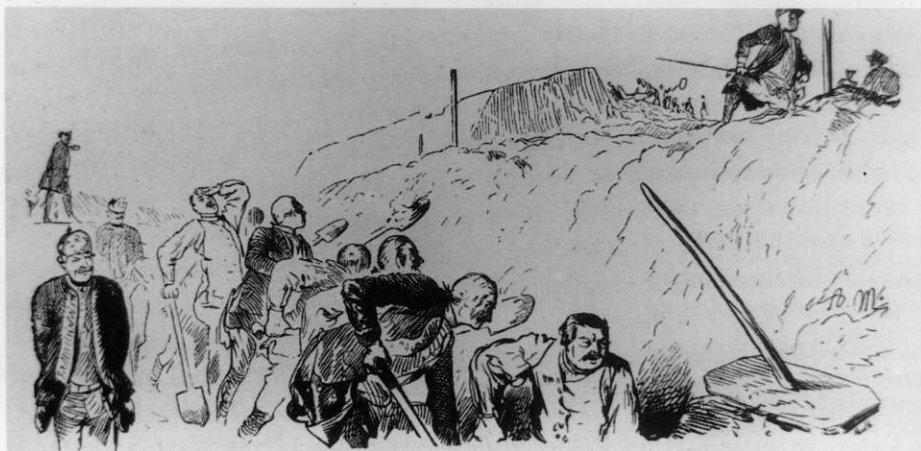
The entrenched camp at Bunzelwitz saved Frederick's army at a critical stage in 1761; this engraving after Menzel shows the ditches under construction, work being supervised by engineer officers (background) and a miner NCO (left).
