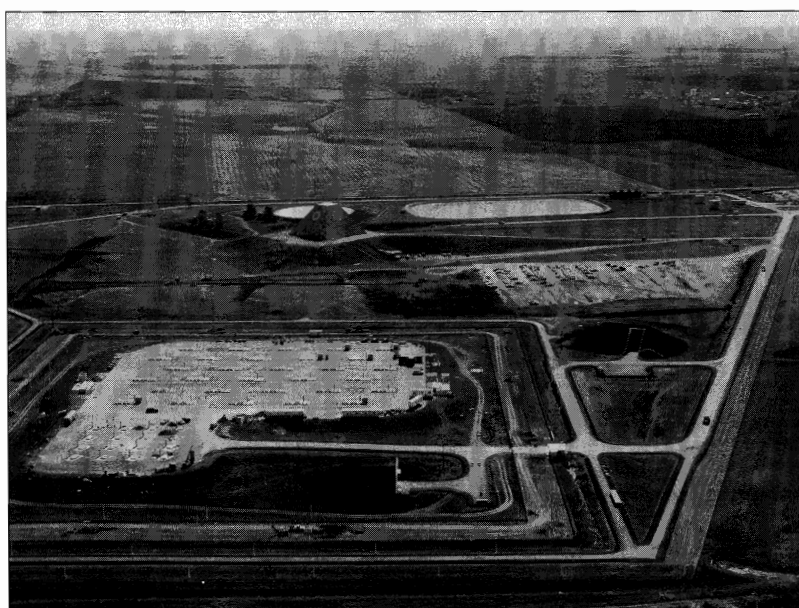
Aerial view of the main missile launch site for the Grand Forks Safeguard site. The Sprint/Spartan launch cells are located in the foreground, the pyramidal Missile Site Radar Building (MSRB) is in the upper center of the photograph. (US Army Space and Strategic Defense Command History Office, Huntsville, AL)
