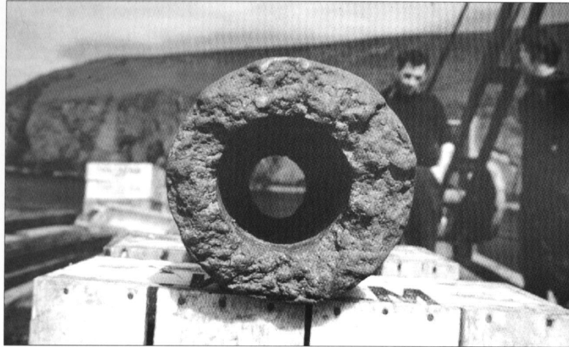
This section of a bronze demi-culverin ( medio-culebrina ) cast with an off-centre bore. A poorly-cast gun would be extremely dangerous to fire. Recovered from the wreck of the Spanish Armada vessel El Gran Grifon , wrecked off Fair Isle off the north of Scotland. (Dr. Colin Martin)
