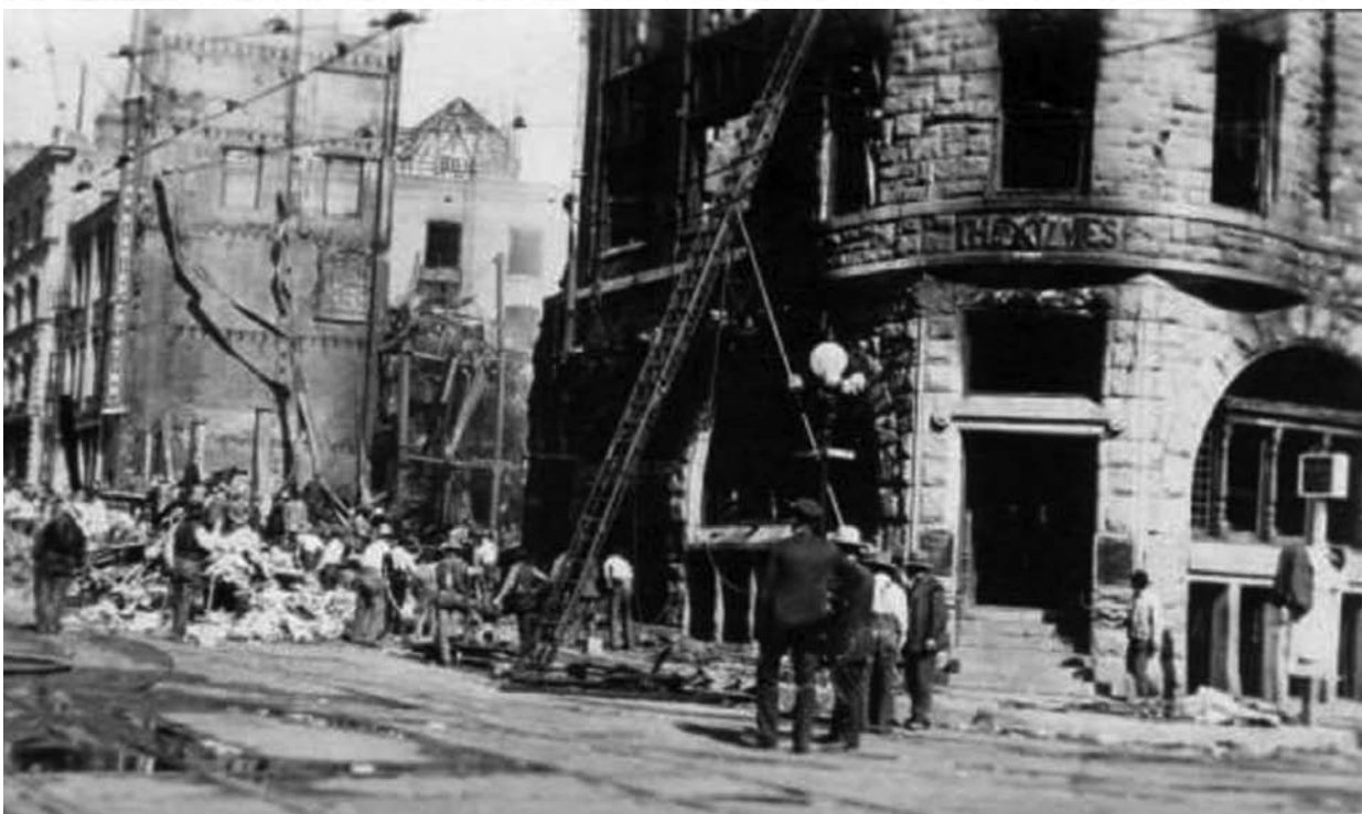
Ruins of the Los Angeles Times Building, 1910.
