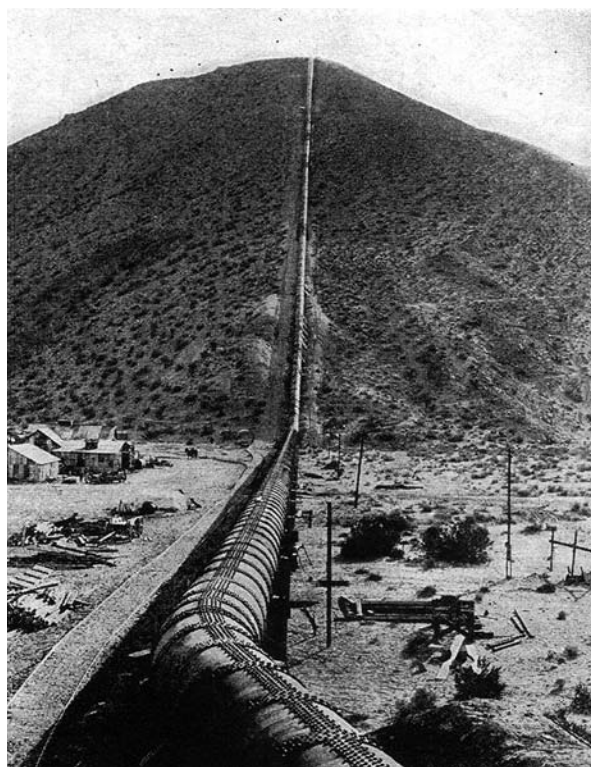
A portion of the Owens Valley Aqueduct.
