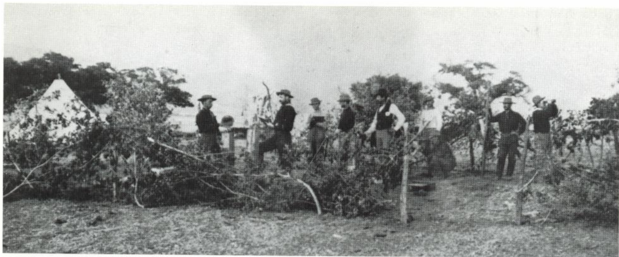
Heliograph Station No 3, Bowie District, Arizona, about 1885, manned by Signal Corps men. In the cloudless south-west, signals could be flashed great distances by mirrors. Both soldiers and Indians used the same communication method (U.S. Signal Corps)
